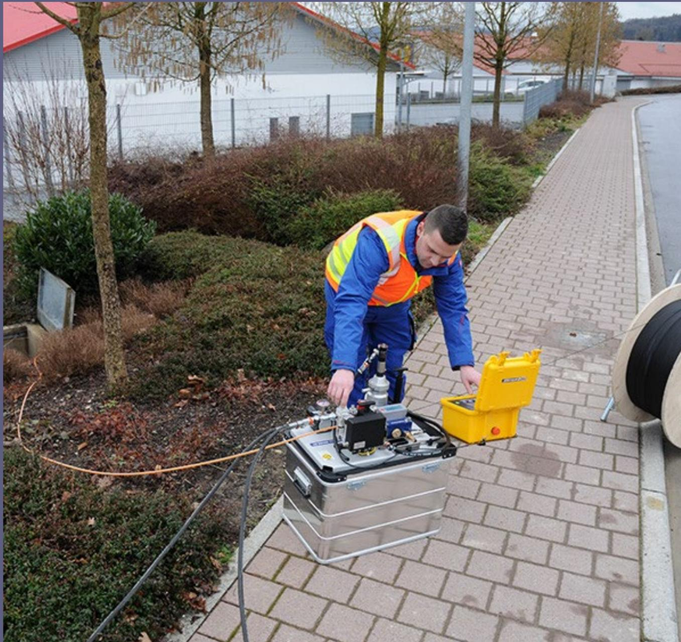
Blowing fiber, also known as jetting, is when a machine is used to float fiber optic cable through the conduit run by using highly pressurized air to push it forward.
