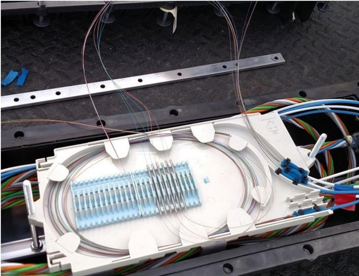
Pistoning is the fibers pushing out of the tubes into the tray and possibly out of the tray too
